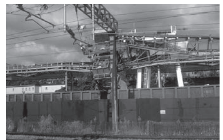
Crossrail: Accident to a rail hopper a week after the Unite members were sacked. Unite stewards say: "This is what happens when you sack safety reps and stewards. Make no mistake this is union busting. It is the sacking of an entire work force to remove the steward and the union off the project".
