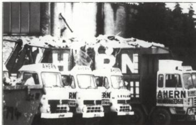
Lorries loaded and ready to leave the site. Waste spills over the top of an unsheeted container: will it end up in the road outside the site?
