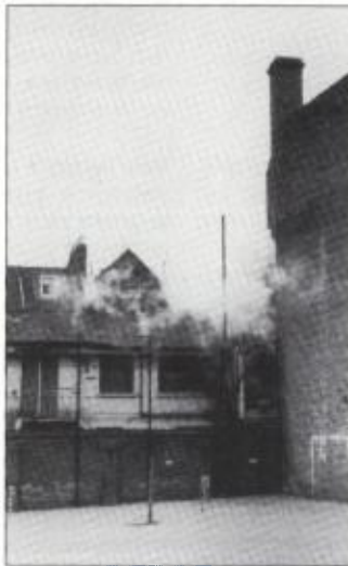
Mystery discharge into school yard.
