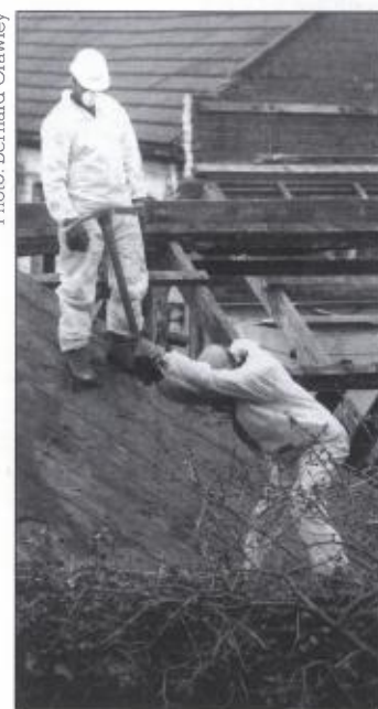
Asbestos roofing removal at the Ascham Street site.
